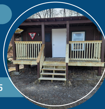
Our Next Renovation: M-05
